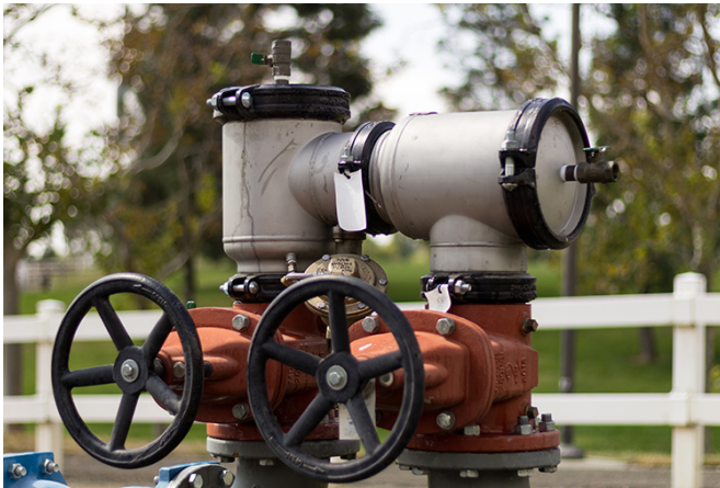
475ST Stainless Steel n-Pattern Reduced Pressure Principle Assembly installed to protect against backsiphonage and backpressure in high hazard applications
