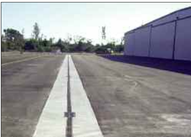
Airport Trench Drain
