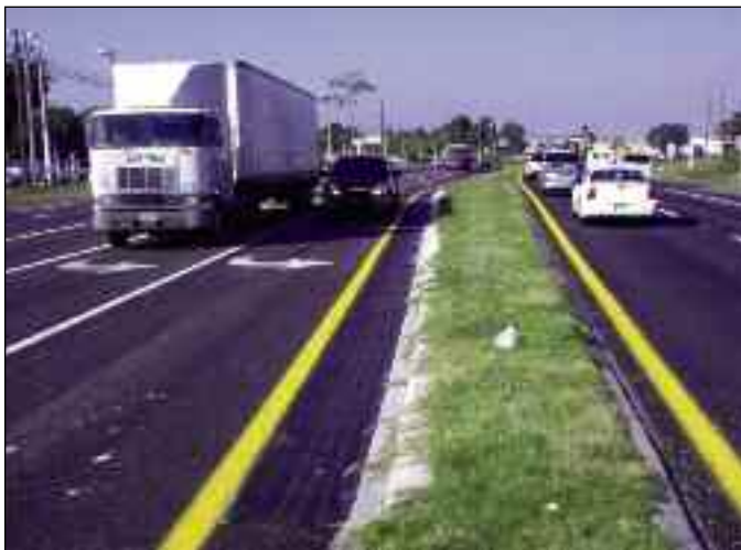
Median Trench Drain
