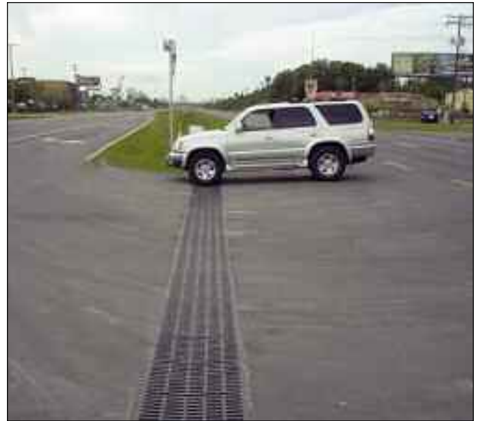
Highway – Z874-FL DOT Grate
