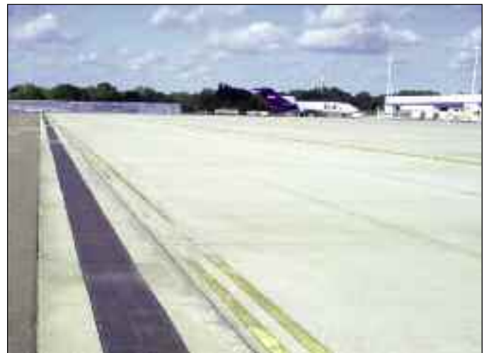
Airport Trench Drain
