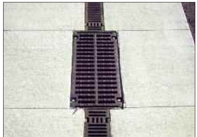
Airport Trench Drain
