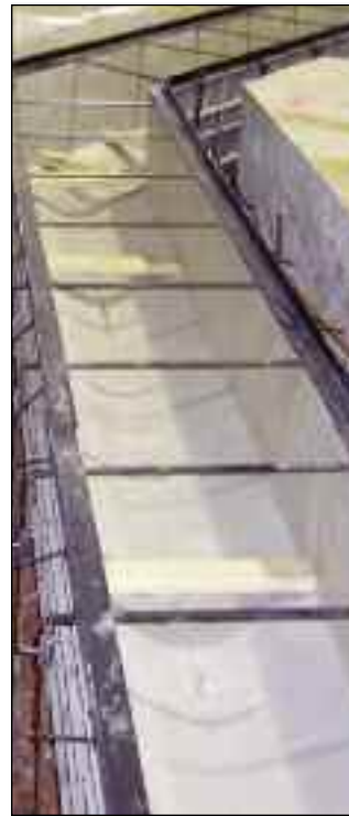
Airport Trench Drain
